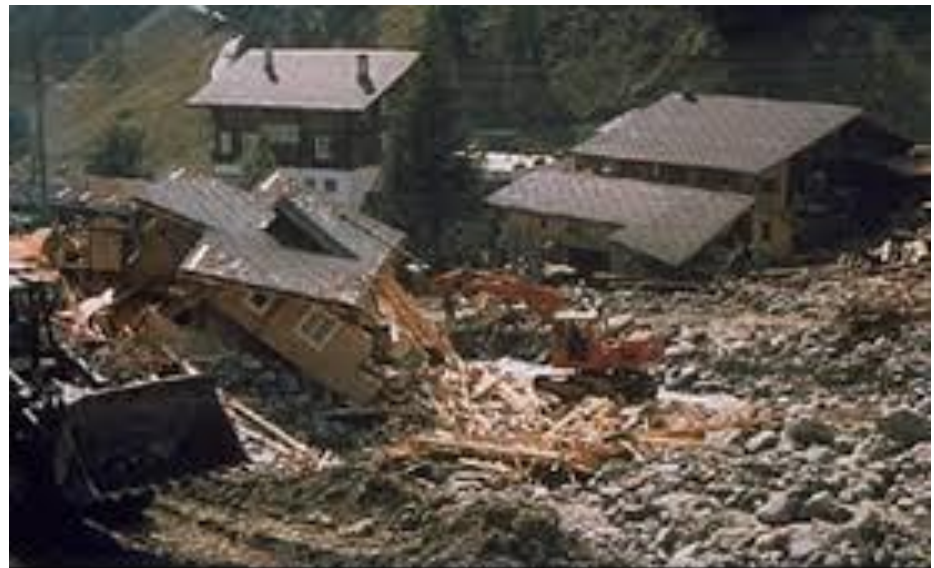
Houses undermined by melting Permafrost
